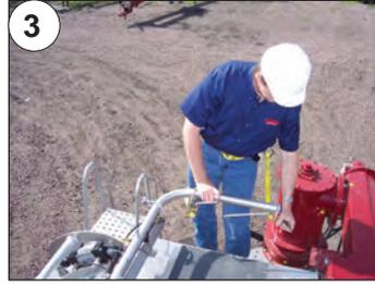
3 Attaching Restraint Straps to the TRAM arm.
